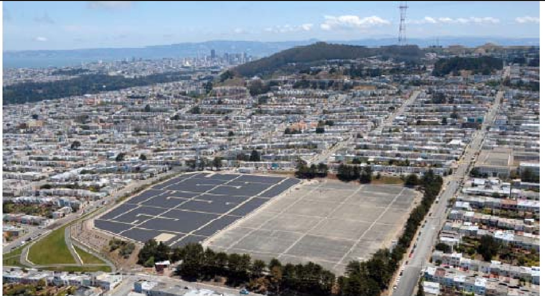
Aerial view of Sunset Reservoir with digital rendering of proposed solar array
